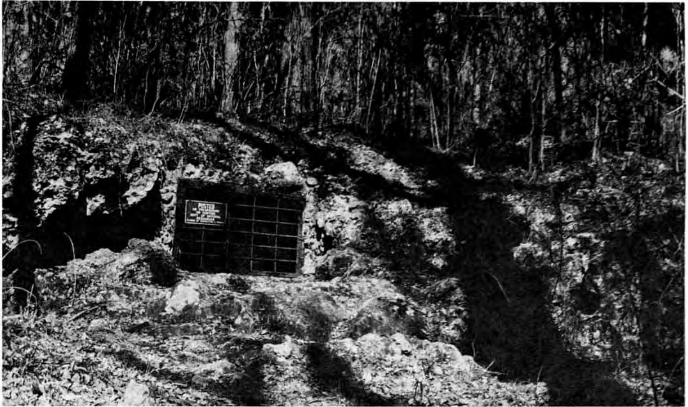
a. Main gate: note cement-filled areas at sides and poorly located sign which restricts air flow. Small entrance size makes increase in predation particularly severe.
