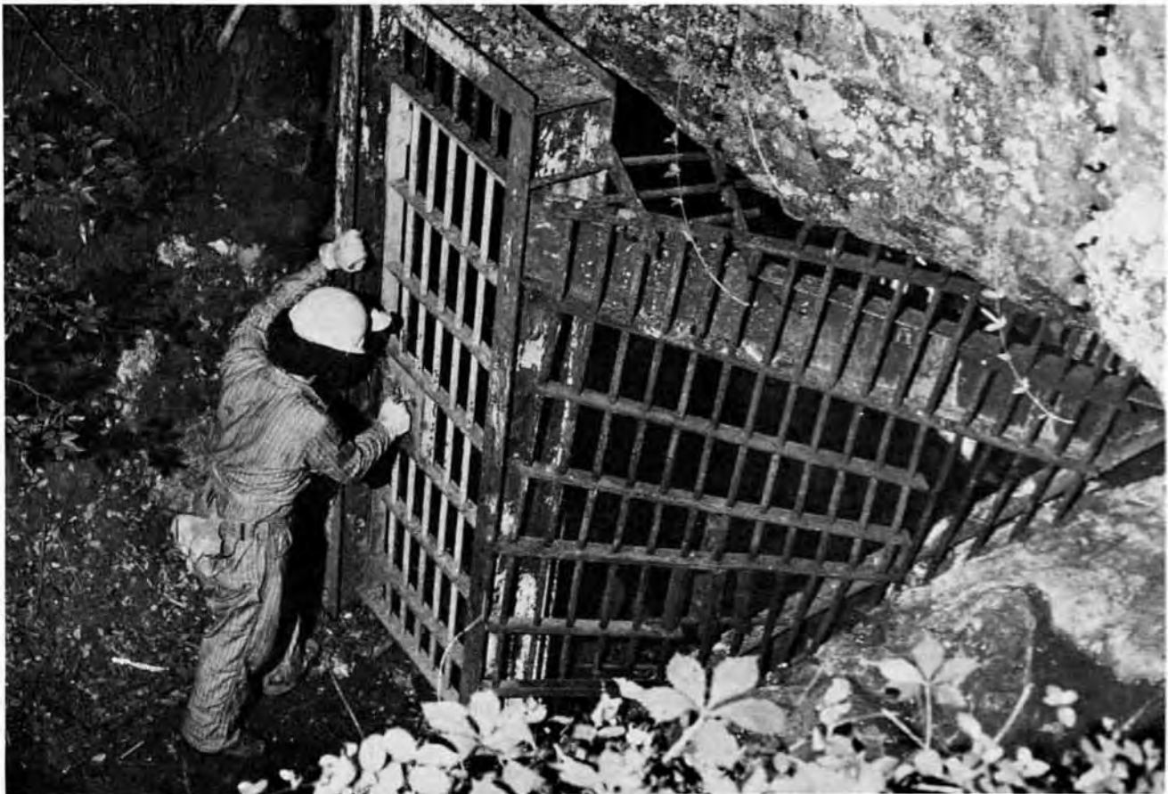
Figure 1—Shelta Cave gate: note the inadequate space between vertical bars and restrictive framing.
